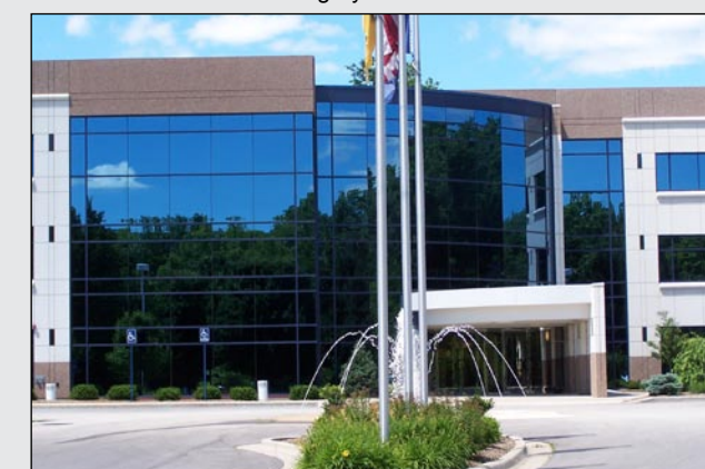
Kenmoor Office Building
