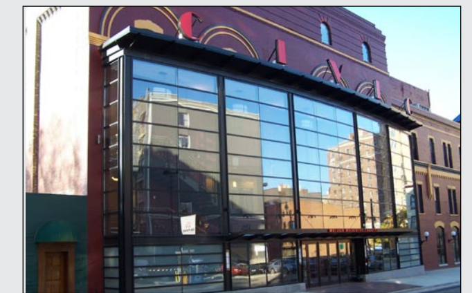
Grand Rapids Civic Theatre Renovations
